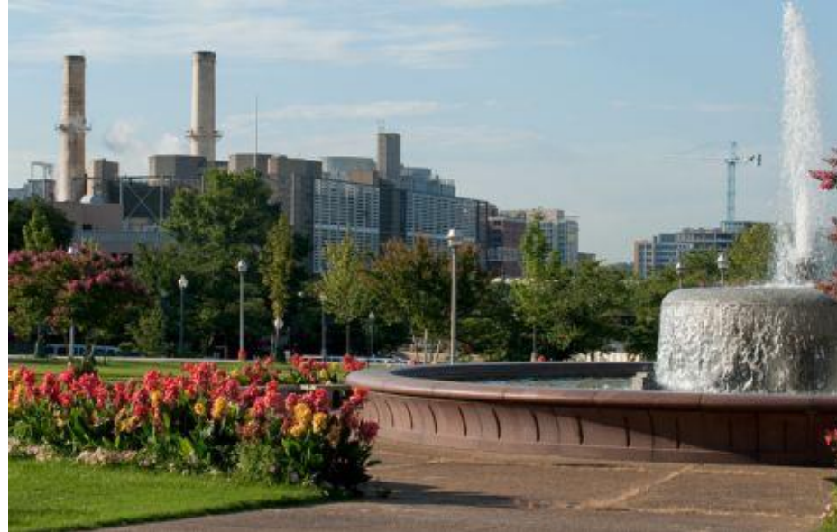
The Capitol Power Plant
